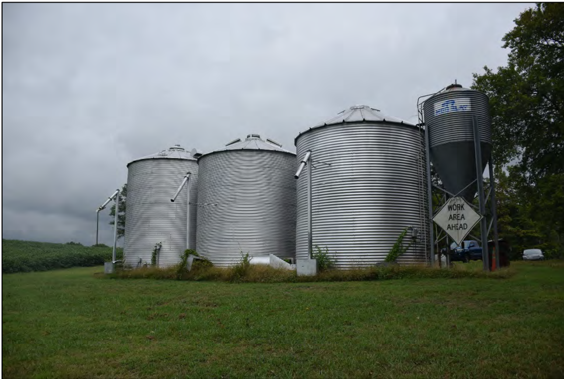
Figure 2.1.49. View of circa-2000 silos, Underwood Farm, facing northwest.
