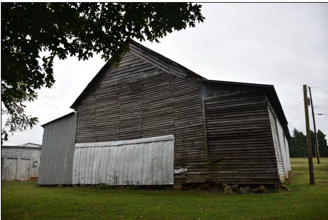
Figure 2.1.22. View of circa-1900 barn, Underwood Farm, facing southeast.
