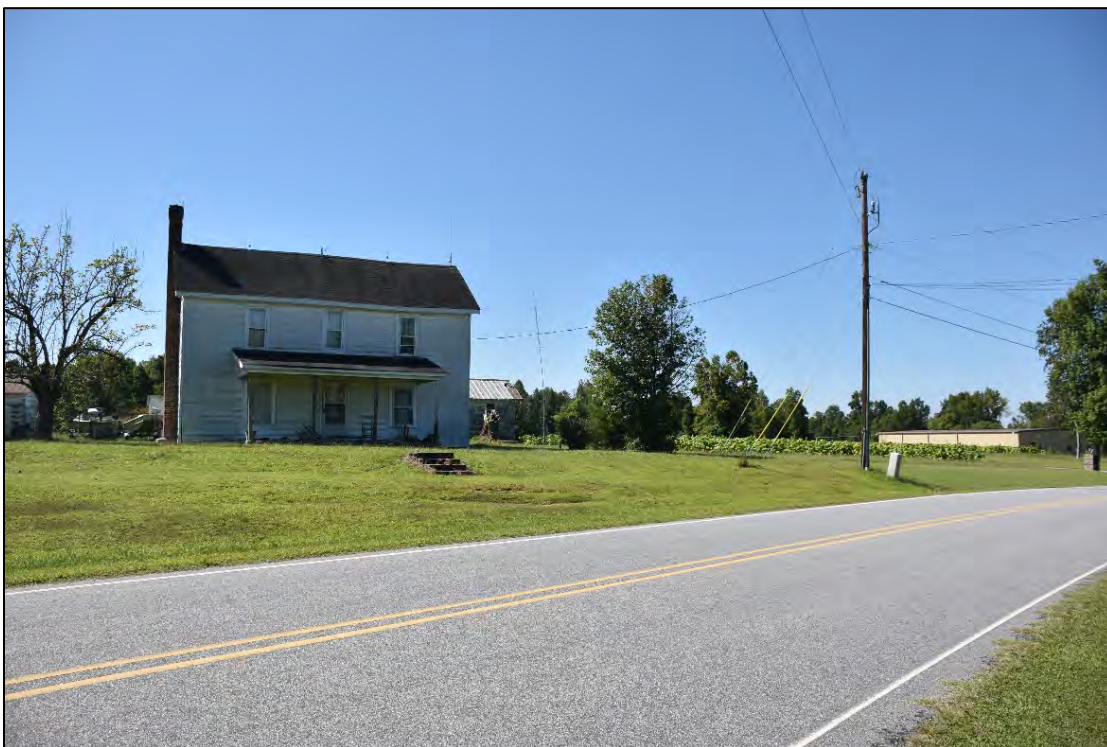
Figure 2.1.58. Welborn House (RD0361), facing south.
