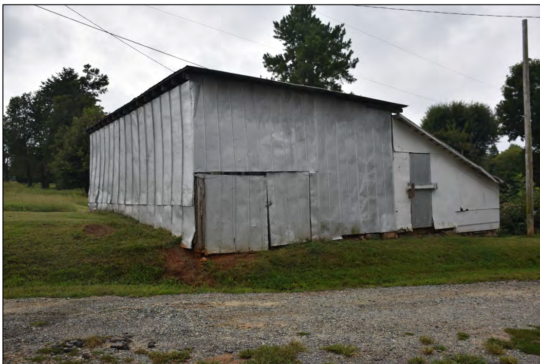
Figure 2.1.32. View of circa-1950 shed, Underwood Farm, facing southwest.
