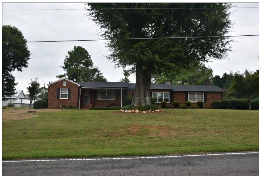
Figure 2.1.12. D. S. Underwood House, circa-1950, front elevation, facing east.
