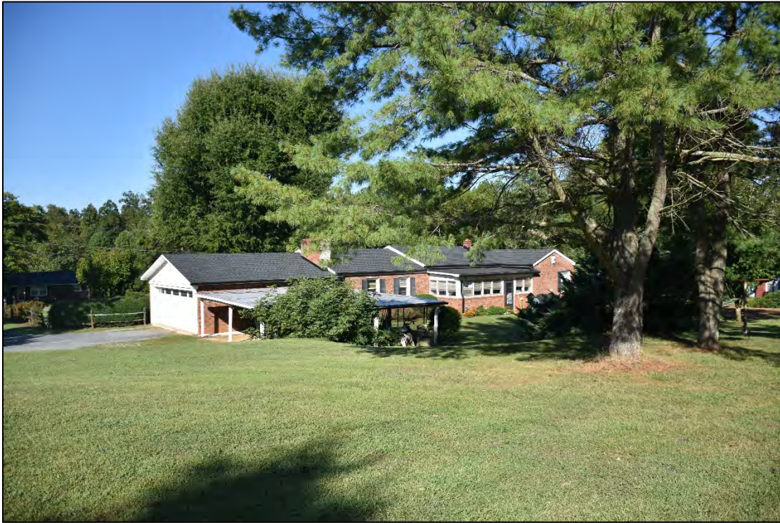
Figure 2.1.15. D. S. Underwood House, circa-1950, rear oblique view, facing west.
