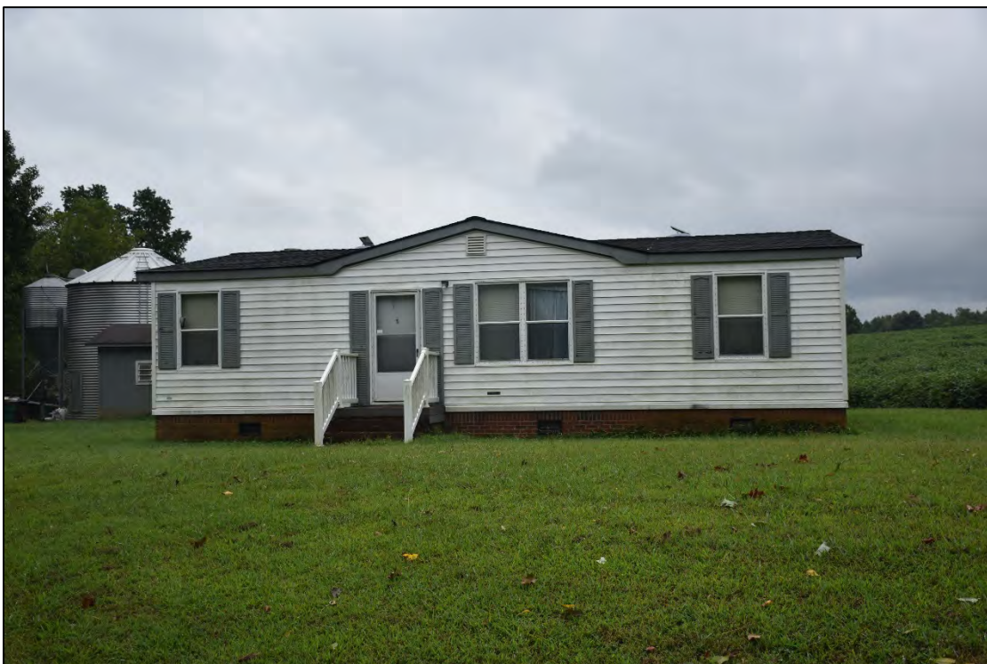
Figure 2.1.50. View of circa-1990 prefabricated home, Underwood Farm, facing south.
