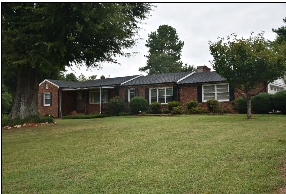
Figure 2.1.13. D. S. Underwood House, circa-1950, oblique view, facing northeast.
