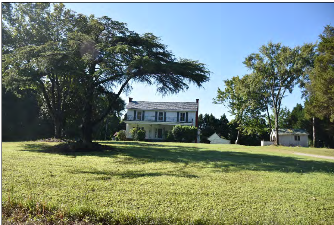
Figure 2.1.63. House and outbuildings, 6219 Welborn Road, facing south.
