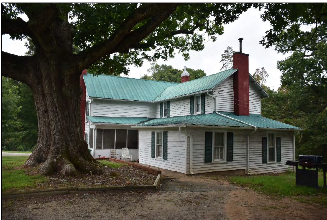
Figure 2.1.10. Underwood House, circa-1880, oblique, facing northwest.
