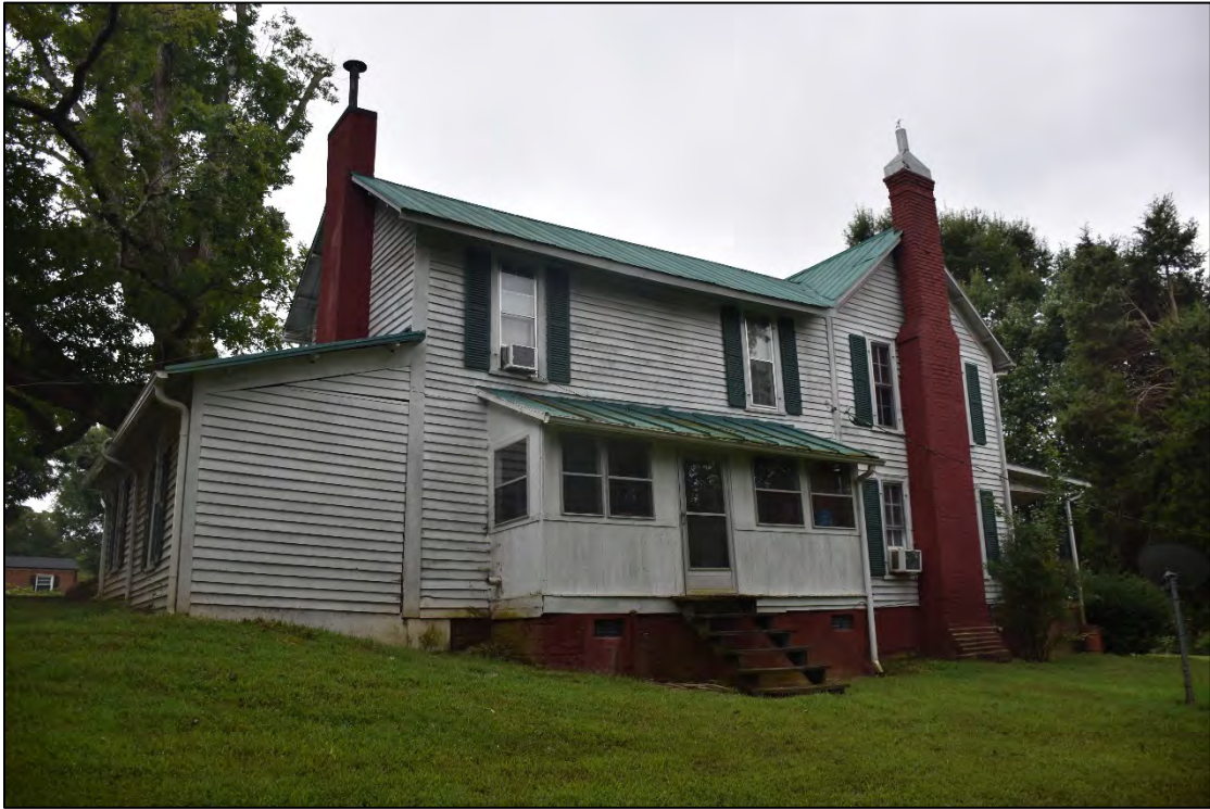
Figure 2.1.8. Underwood House, circa-1880, north elevation, facing southwest.
