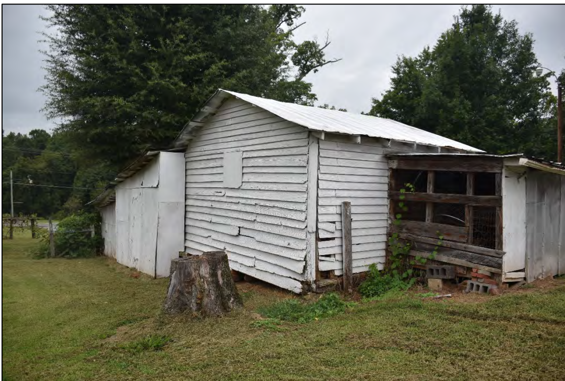
Figure 2.1.31. View of circa-1930 shed, Underwood Farm, facing west.
