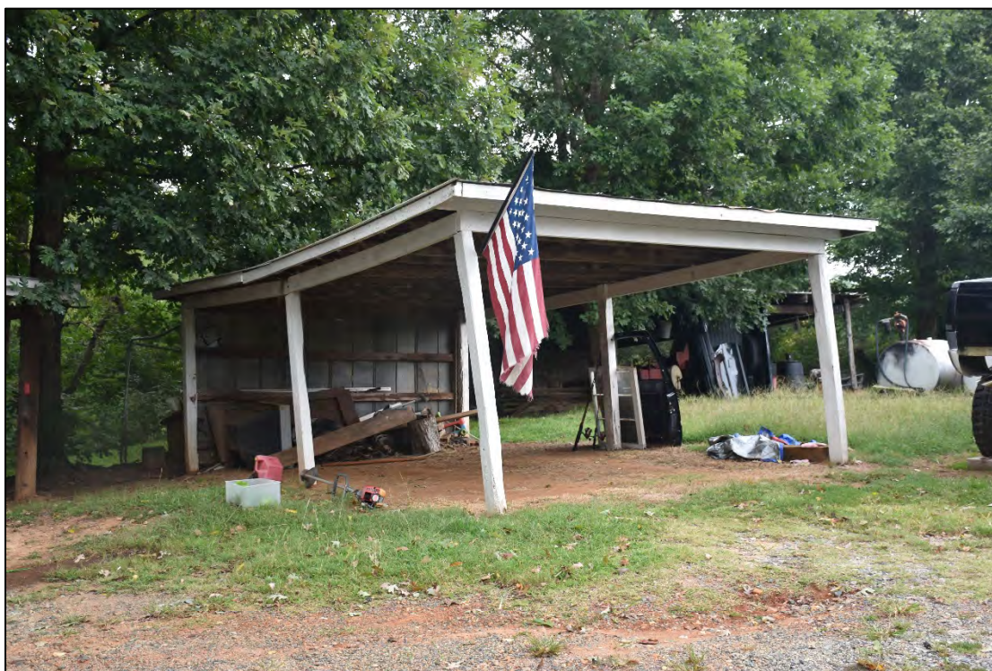
Figure 2.1.18. View of circa-1950 open storage, Underwood Farm, facing north.
