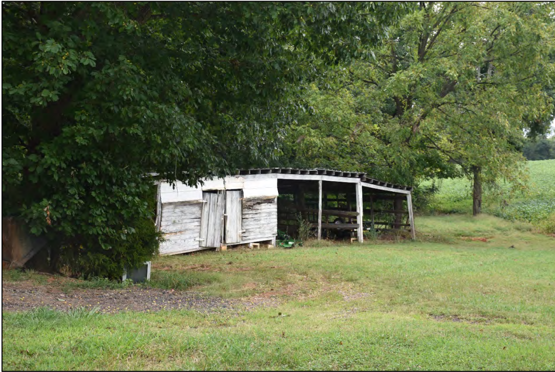
Figure 2.1.45. View of circa-1960 shed/storage building, Underwood Farm, facing southeast.
