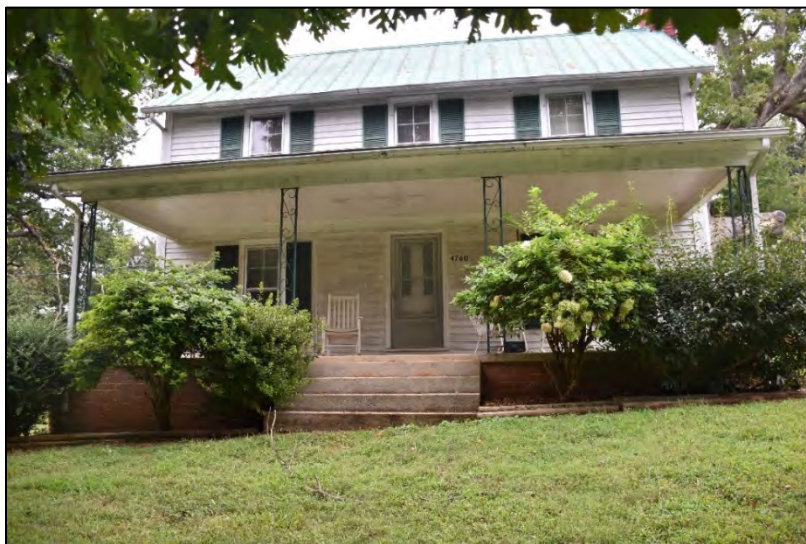
Figure 2.1.5. Underwood House, circa-1880, front elevation, facing northeast.
