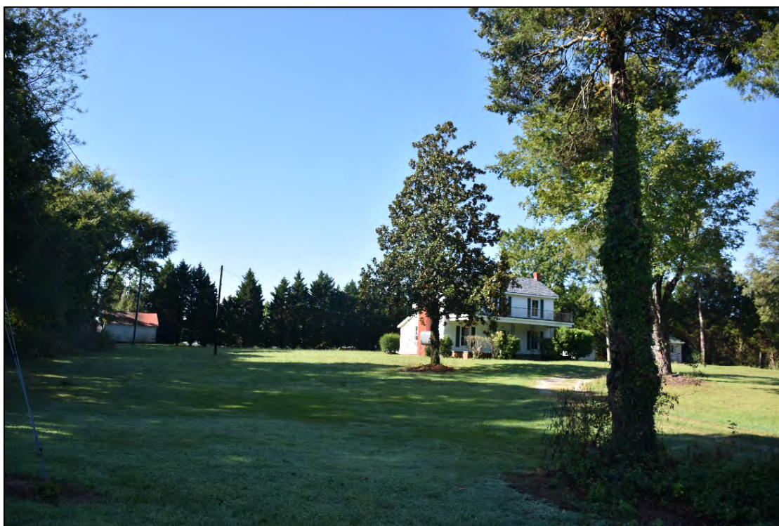
Figure 2.1.64. House and outbuildings, 6219 Welborn Road, facing south.
