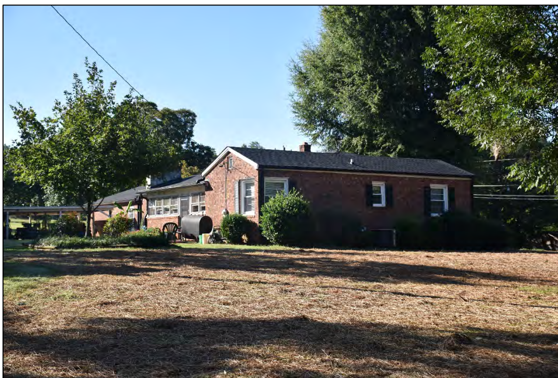
Figure 2.1.14. D. S. Underwood House, circa-1950, north elevation, facing south.
