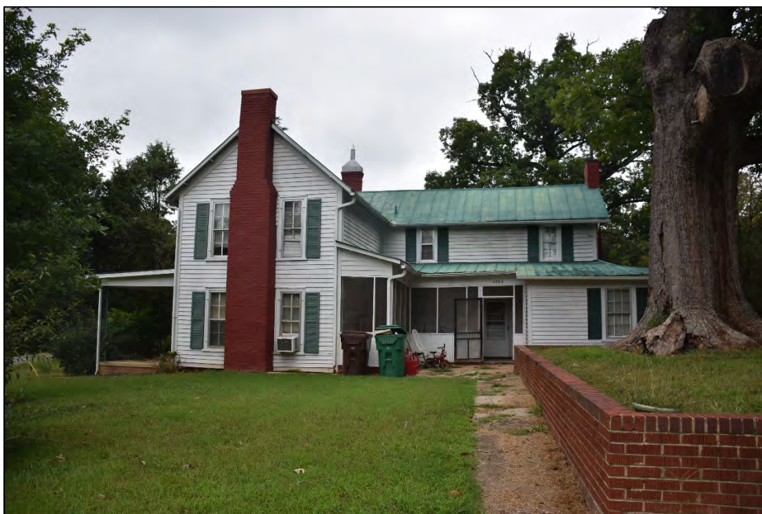
Figure 2.1.11. Underwood House, circa-1880, south elevation, facing northwest.
